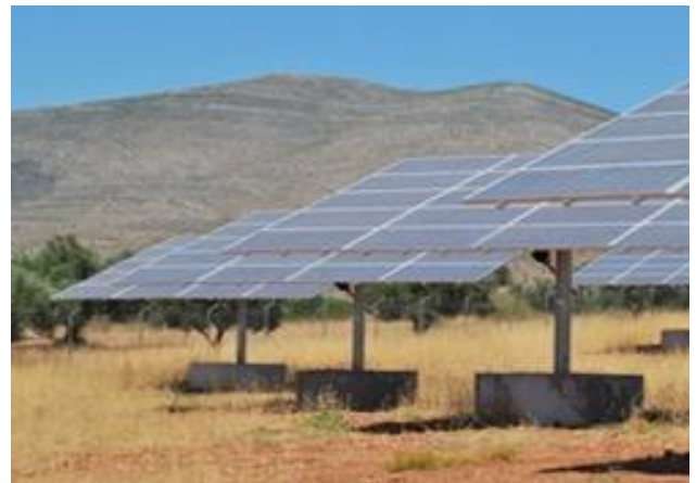
Helida1 99.68 kWp (dual axis)
