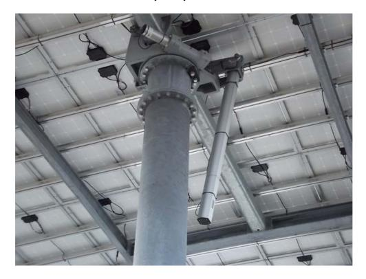
Compared to the previous elevation motor the new EMO no longer uses a harmonica type cover. Now the EMO is a complete closed system, by what the intrusion of dirt and water will be avoided and the life-cycle of the motor will be significantly increased.
